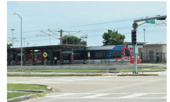
METRORail Train at Fannin South Transit Center
